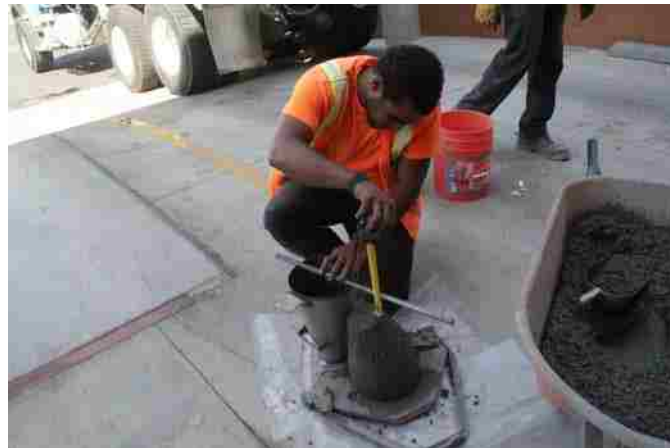
Figure 7- Slump Measurement by ACI Technician
