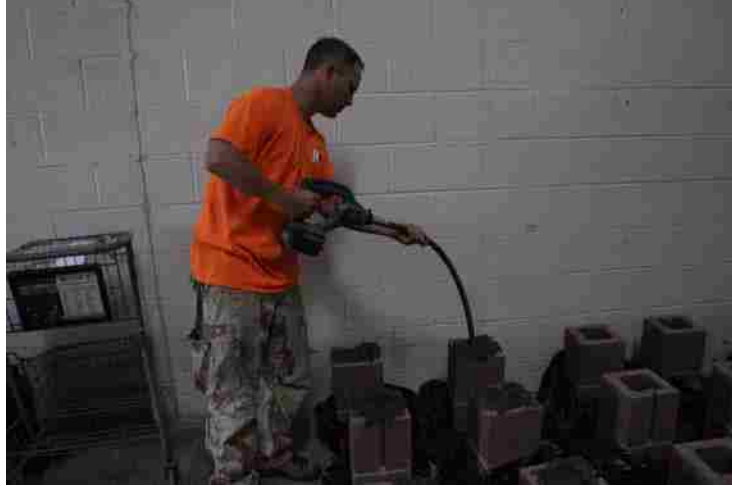
Figure 4- Consolidation of Grout
